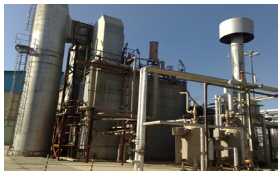
Fig. 1. The Steam generator of oil refining company of Kermanshah
